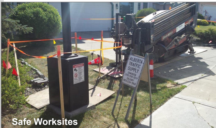
Snow fence around larger excavations
