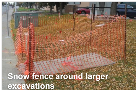
Secure and covered excavations
